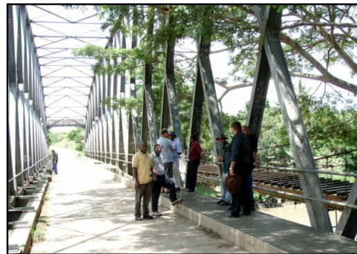
Plate 5 Detail of bridge with the old bridge to right.
